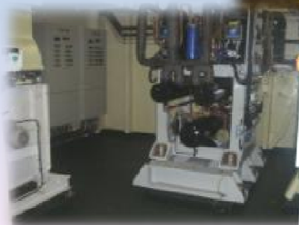
Anti shock digital Scroll compressor unit
